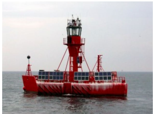
Liverpool's modern Mersey Bar Light Float
